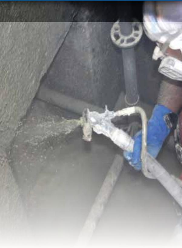
The Graco M680™ Mortar Pump handles abrasive materials such as epoxy mortars, non-skid coatings or cementitious materials, and tackles difficult polymers with fillers such as glass flake, silica or sand.
